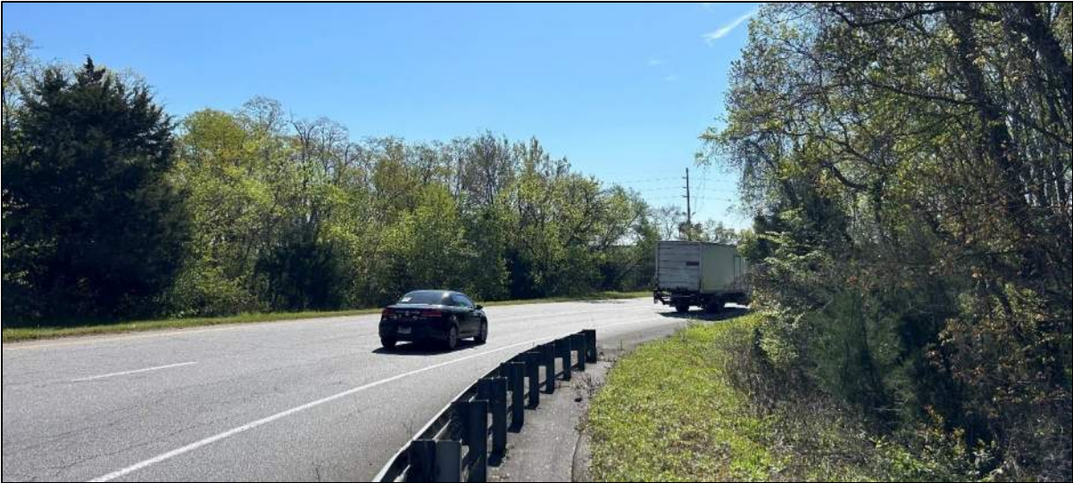
Figure 6: View along the NB Off-Ramp approaching E. President Street
